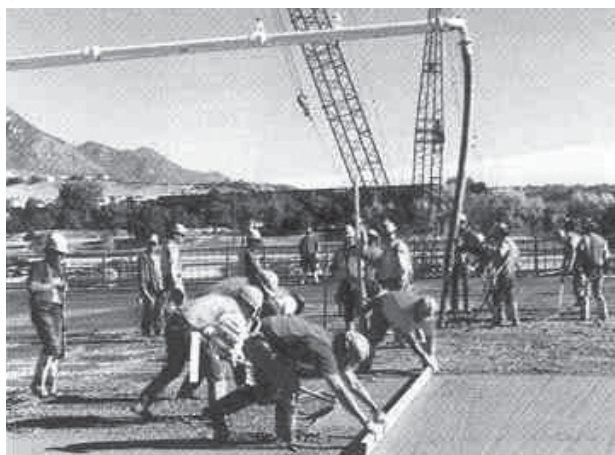
Finishing Concrete Flatwork
