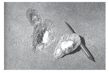
A popout is a small fragment of concrete surface that broke away due to internal presssure, leaving a shallow, typically conical, depression.
