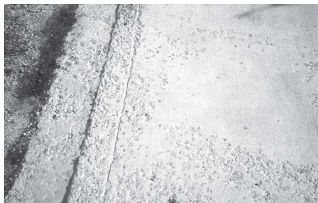
Scaling concrete surface
