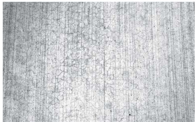
Crazing Concrete Surface (Dampened)
