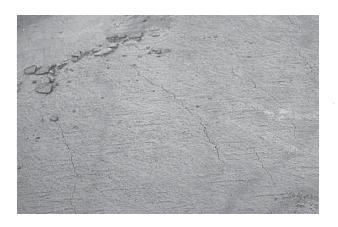
paste shrinks during early hydration which produces very small micro cracks. When the rate of evaporation is high and the concrete has enough strength (or stiffness) to cause horizontal shrinkage the normal micro cracking tendency is accentuated and noticeable plastic cracking may result.
